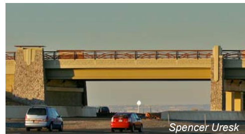
Bridges are a mix of colored concrete with stacked stone accents and an artistic railing depicting blade of grass. Overpasses are lower than typical highways to minimize their apparent scale.
