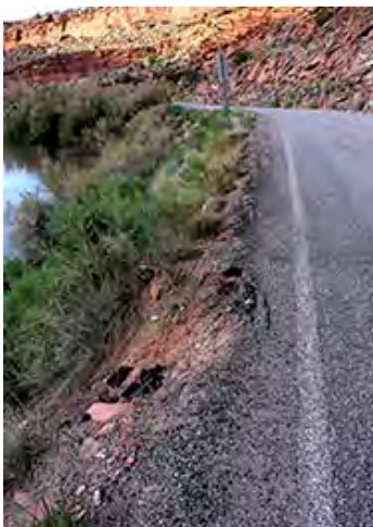
Many sections of SR-128 lack clear zones and railings
