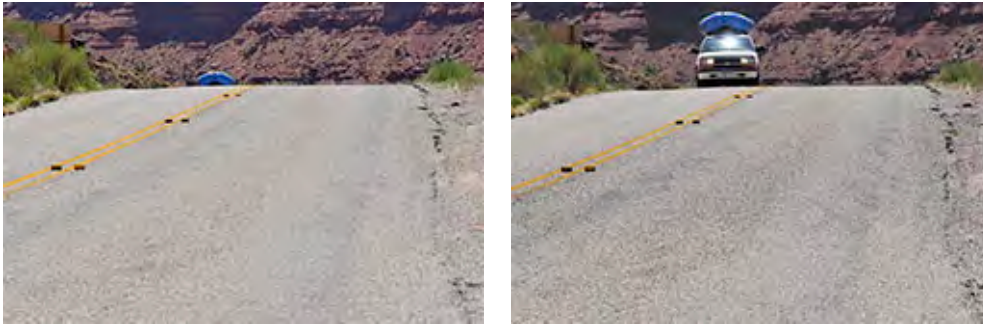
Abrupt vertical curves, such as this on SR-128, can hide oncoming traffic
